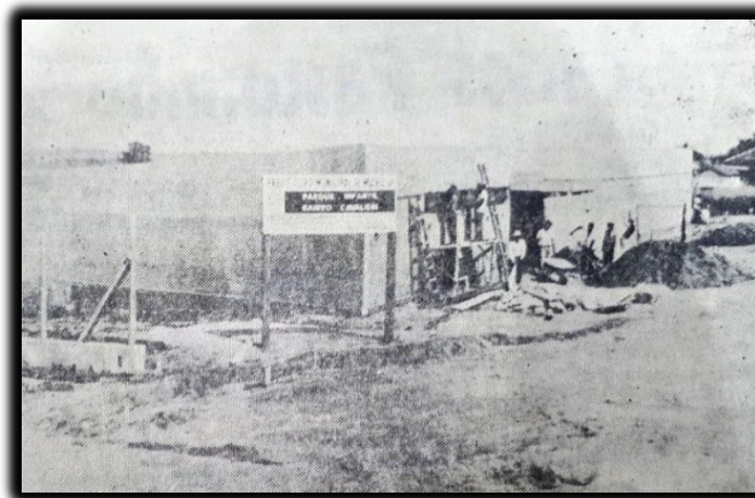
Figure 6 – Construction of the “Walt Disney” Kindergarten
